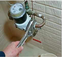
When loosening/disconnecting the supply line, be sure not to strip the connection. Once it is disconnected, it is strongly recommended that you properly install a cap on the water meter side of the disconnection to prevent any possibility of leaks.
